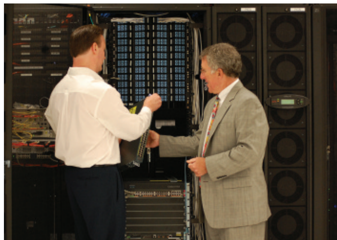
ChimeNet Data Center
